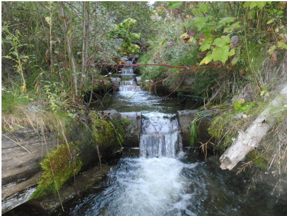
Six log weirs on Mill Creek (Smith property) upstream of box culvert.
