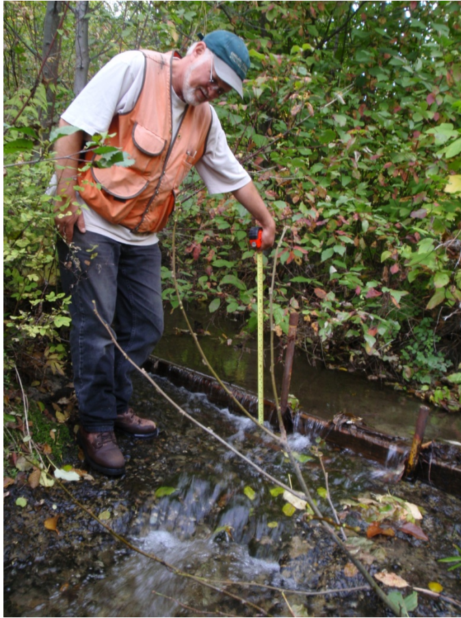
Diversion structure on Mill Creek (Smith property) at head of log weirs. Alan is standing on a chipped slab presumed to be part of historic dam.
