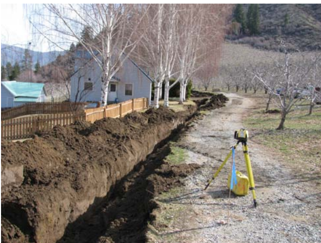
Mountain West controls excavation to sub-grade elevation.
