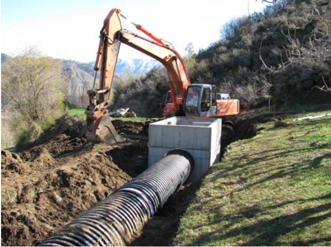
Connection of 36-inch pipe to flow control structure. Interior control gates installed.
