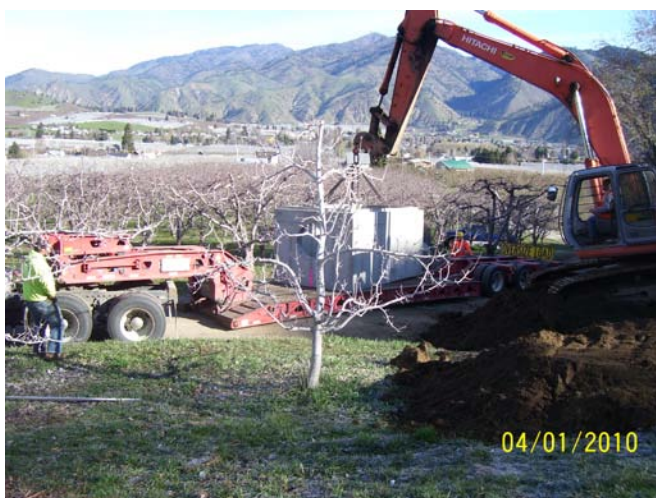
Delivery of flow control structure at Sta. 69+45.
