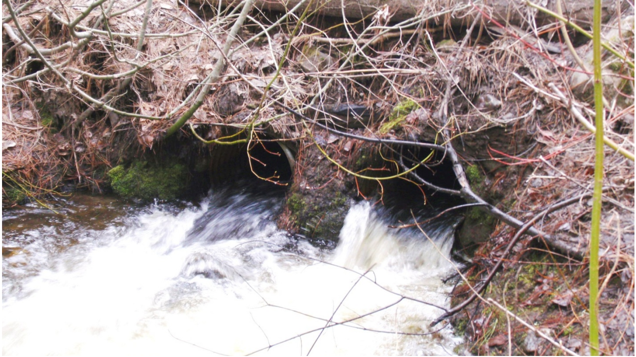
Photo 1. Coulter Creek barrier culvert/s 36" squash pipe and 18" relief culvert - looking upstream
