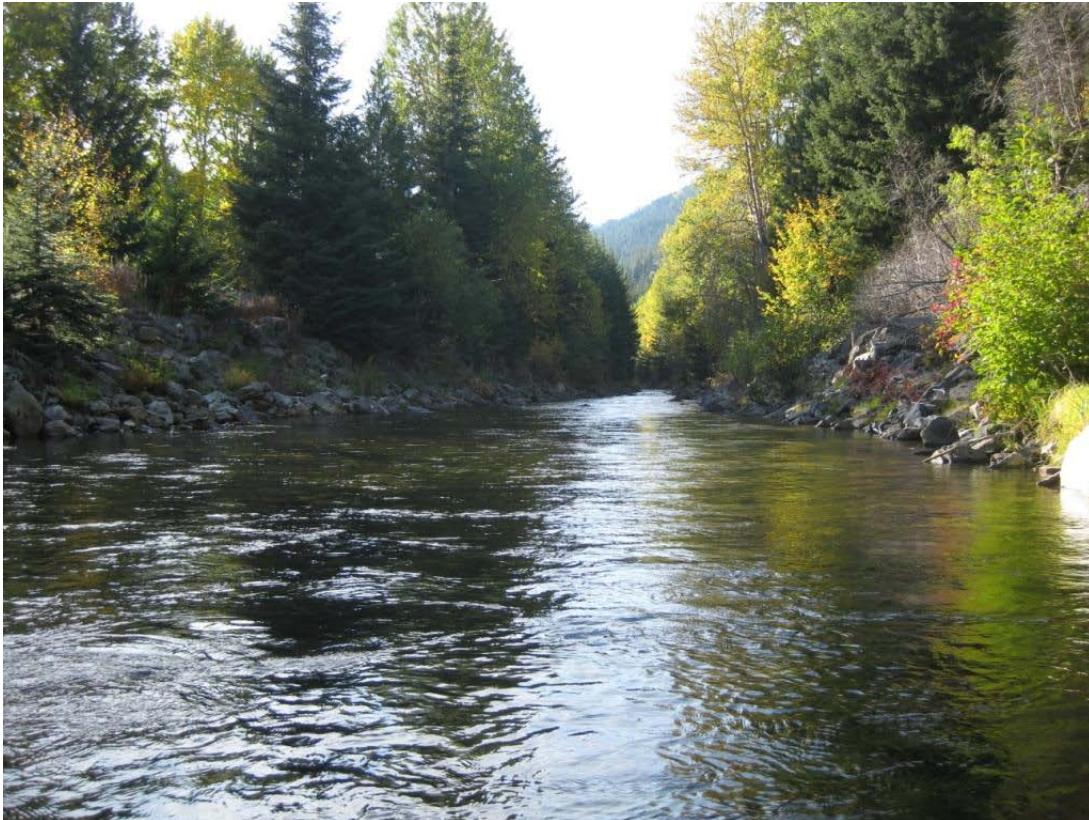
Figure 5. Typical view of the Dire Straits Project Area. Notice the rip rap that dominates the stream banks through this segment. The railroad grade is located to the left and the dike that protects the PUD lines is located to the right.
