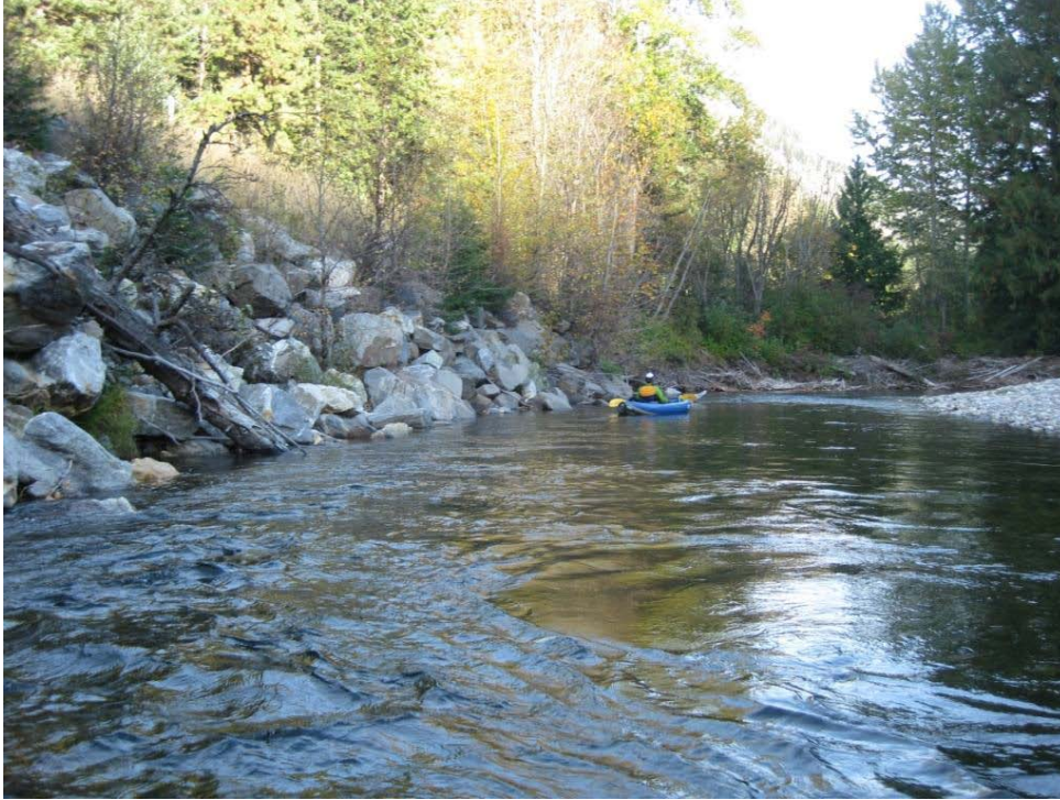
Figure 19. View of rip rapped section of project area 3 along the north bank of US Highway 2. Notice the lack of riparian vegetation and large wood through this section of channel.
