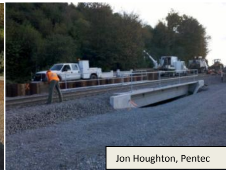
Image 4. Photos showing construction of trestle bridges under the new line of BNSF railroad track in Edmonds, WA. Photos range from August 2010 to early October 2010.
