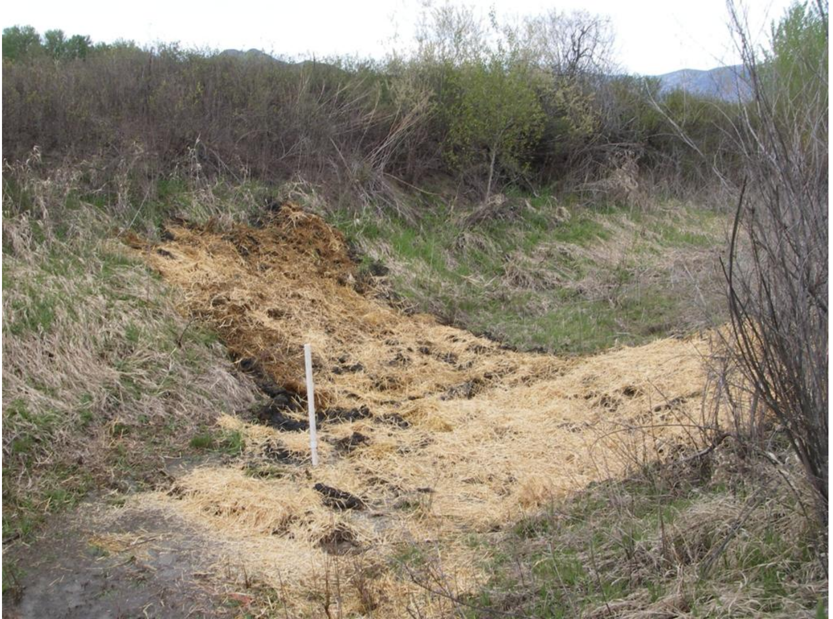
Restored west/Similkameen test well with piezometer.
